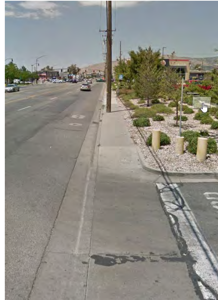
Figure 29 - Narrow Sidewalk with Obstructions along 300 West
