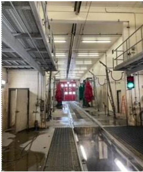
Figure 1 - Jordan River Service Center Wash Bay
