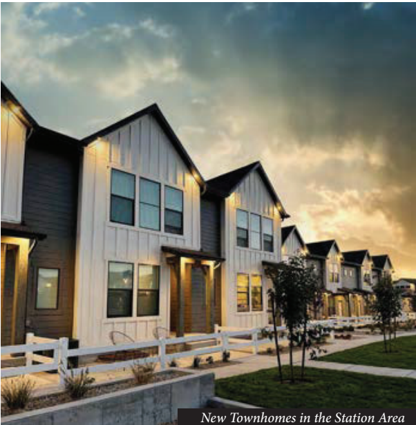
New Townhomes in the Station Area
