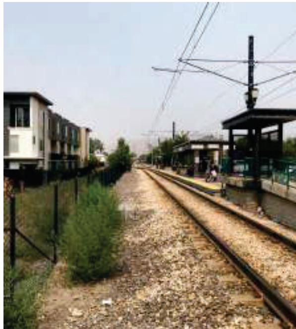
Current view of west-side access to the TRAX platform / GSBS Consulting
