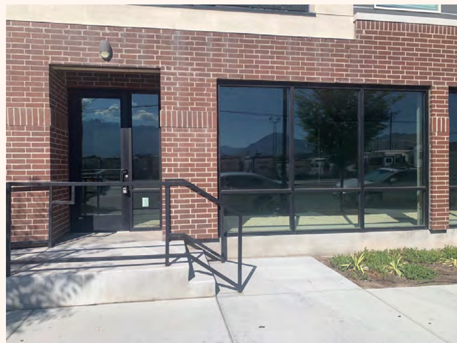
This storefront is an example of what future mixed use should not aspire to. The railing and height above the sidewalk cuts off the storefront to the pedestrian realm. The storefront are also the same throughout the building and does not offer opportunities for businesses to bring their merchandise onto the pedestrian realm or distinguish themselves from the other businesses adjacent to them. Areas for increased signage are also limited to the windows, cutting off sightlines of the street or the business merchandise.
