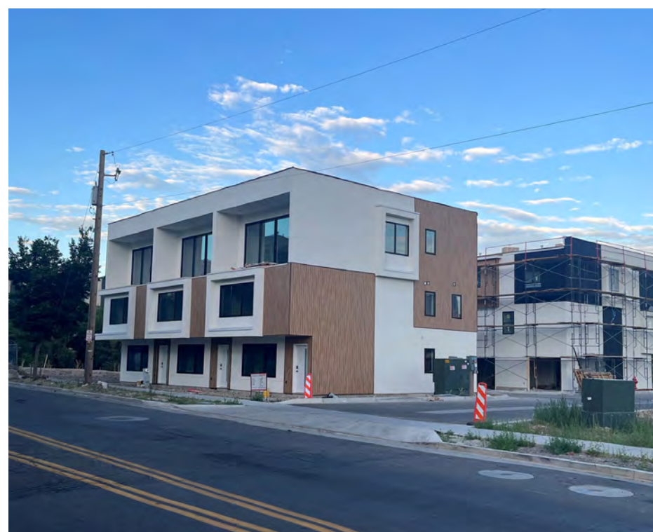
FIGURE 2.5: HOUSING UNDER CONSTRUCTION ALONG MAIN STREET
