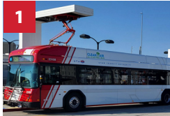
Meadowbrook Bus Charging Infrastructure
