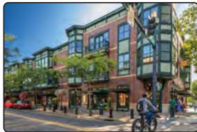
Example of two stories of residential over retail
