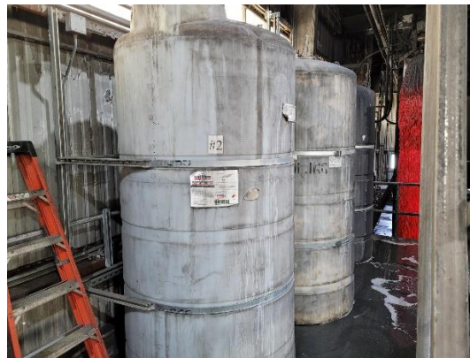
(Figure 3- Warm Springs Alkaline Soap Tank)
