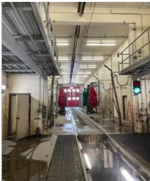
Figure 1 - Jordan River Service Center Wash Bay
