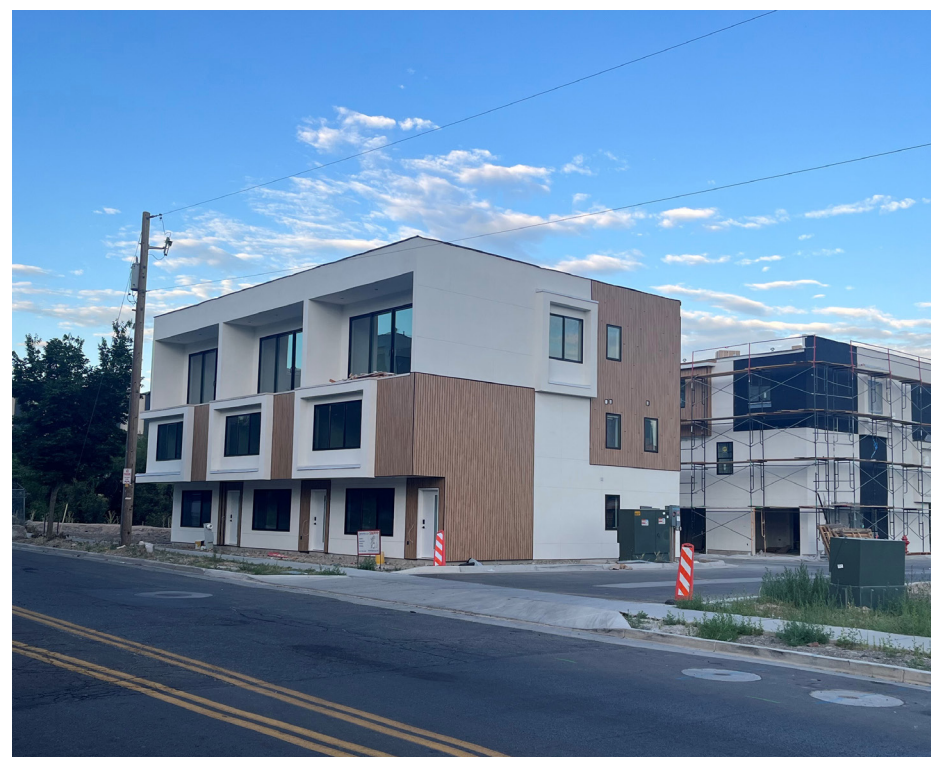
FIGURE 2.5: HOUSING UNDER CONSTRUCTION ALONG MAIN STREET
