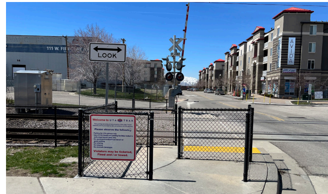
EXAMPLE BARRIER AT THE INTERSECTION OF FIRECLAY AVENUE AND THE TRAX LINE
