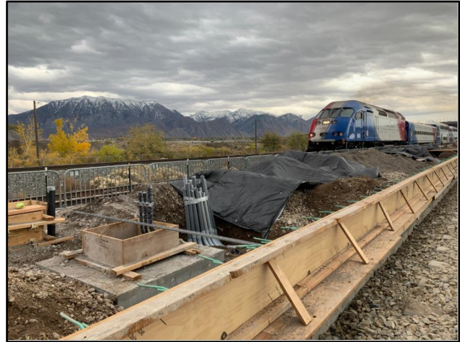
Pictures from 10/26- Station Platform forming occurring. Some foundations have been poured
