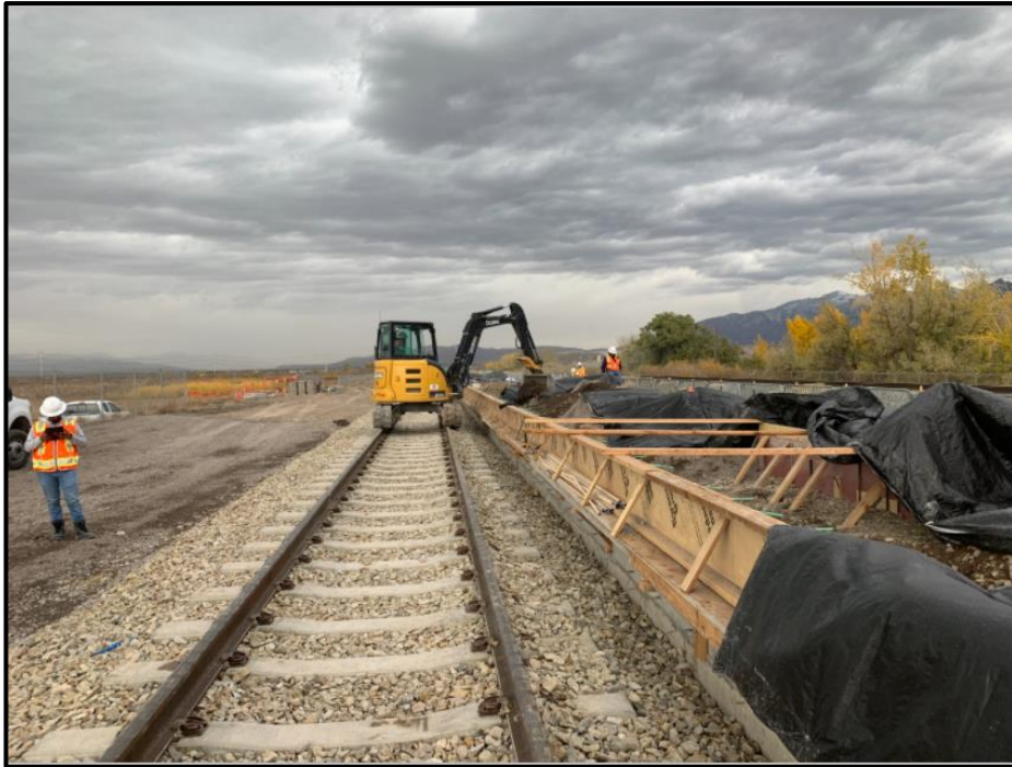
Pictures from 10/26- Station Platform forming occurring. Some foundations have been poured
