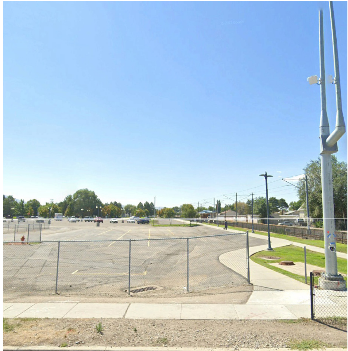
Figure 3.9 Existing Parking Lot Near Fort Union Station on 7200 South
