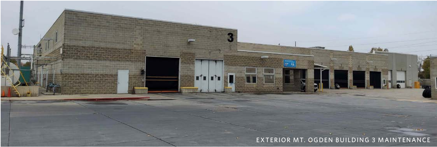
Mt. Ogden building 3 serves the maintenance needs of the current Mt. Ogden bus fleet, including battery electric buses for OGX. Facilities maintenance and road crew also utilize this facility.
