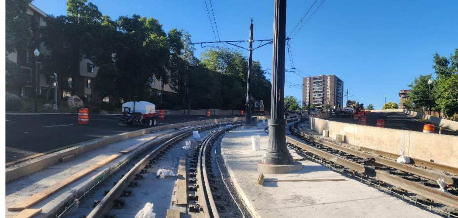
RESTRAINING RAIL INSTALLATION
