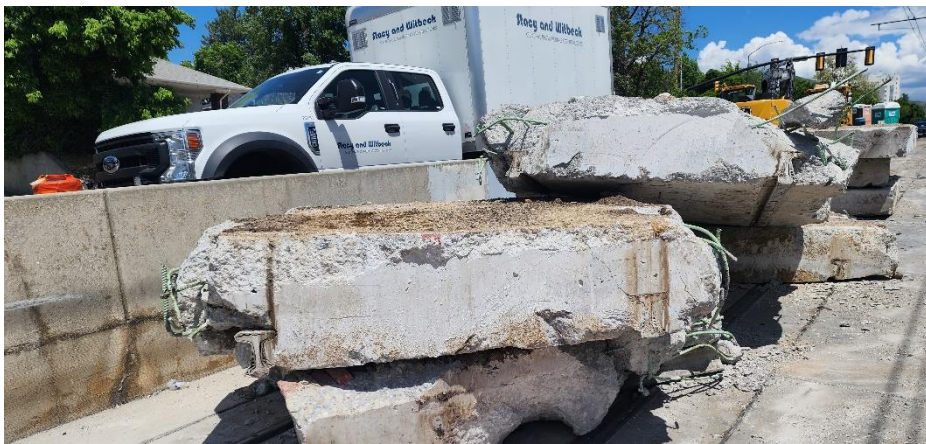
REMOVAL OF OLD TRACK SECTION
