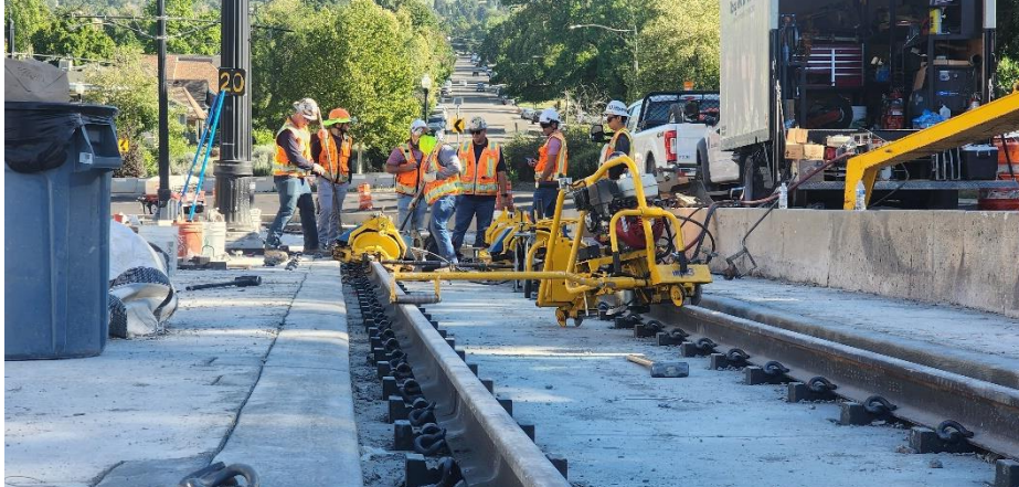
FINAL WELDS AND DESTRESSING
