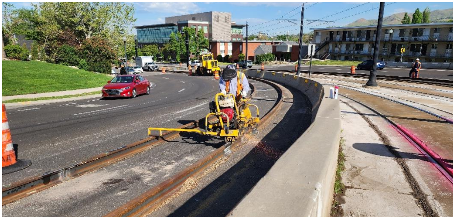
PRE-WORK: STAGING & WELDING
