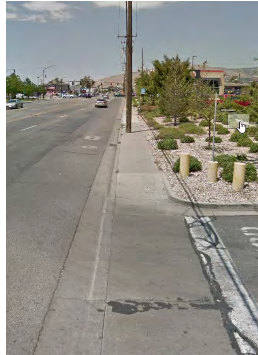
Figure 29 - Narrow Sidewalk with Obstructions along 300 West
